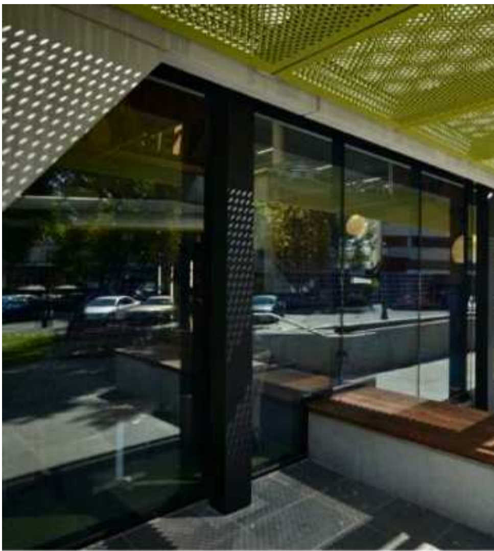
WIN 01: GENERAL GLAZING AND INTEGRATED LOUVRE SYSTEM
